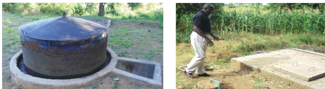
Figure 13 A floating drum bio-digester in Matinyani Kitui County. Right: A fixed-dome model
