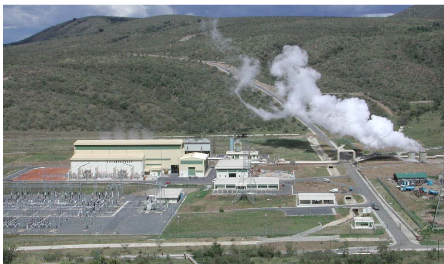
Figure 24: Olkaria II Geothermal Power Station (Flash Steam Power Plant)
